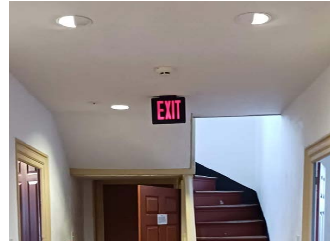
143-1: Existing egress signage at the first floor hallway.
