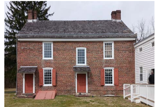
21-1: South facade with two doors; the door on the left leads directly to Room 103.
