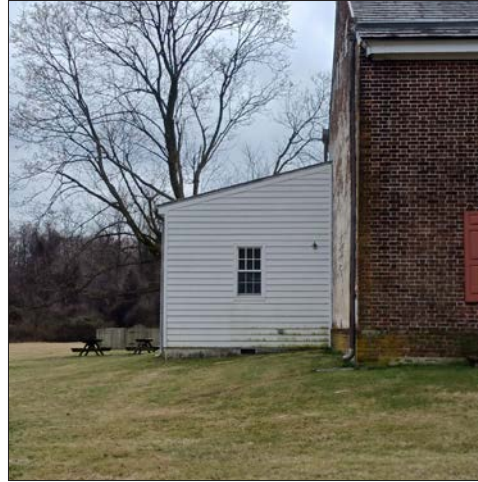
39-4: The 1990s addition is in good condition though moss is growing on the vertical surfaces.
