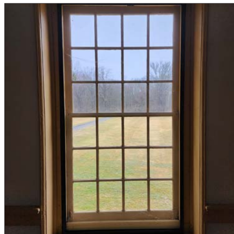
98-4: Window frame is original, sash and storm window date to 1999.
