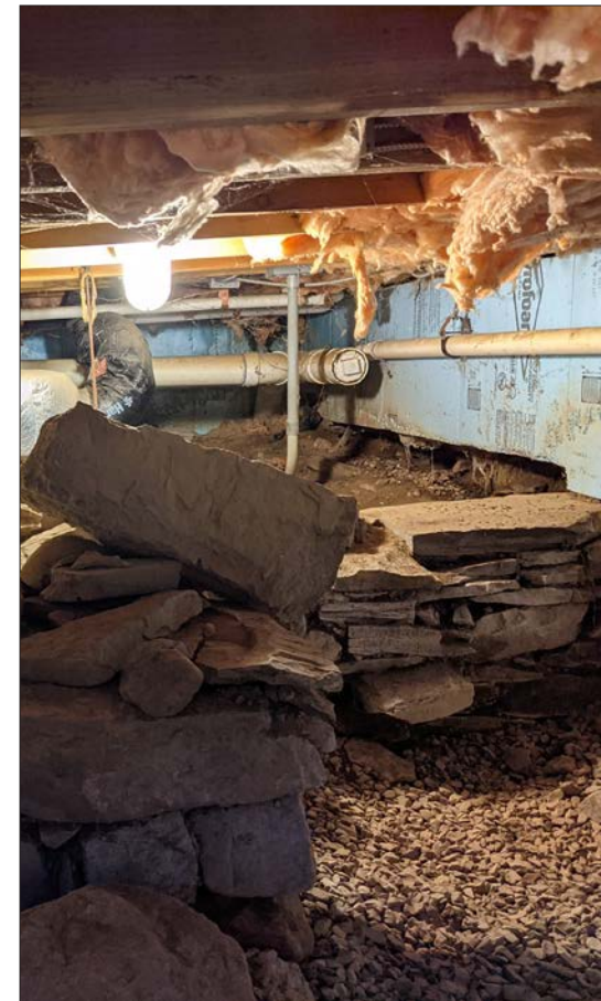
23-1: Stone wall underneath the addition.
