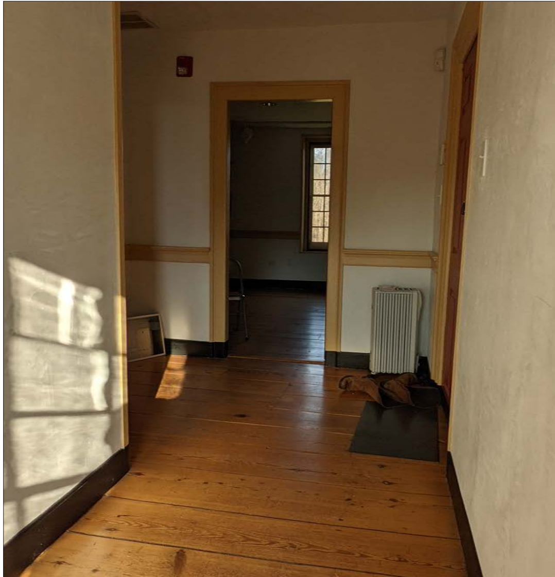
87-1: Overview of the second floor landing looking towards interior.
