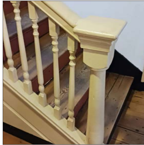
68-4: Baluster and railing.
