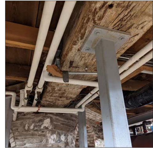
59-3: Structural columns supporting wood beam; structural steel added after 1990.
