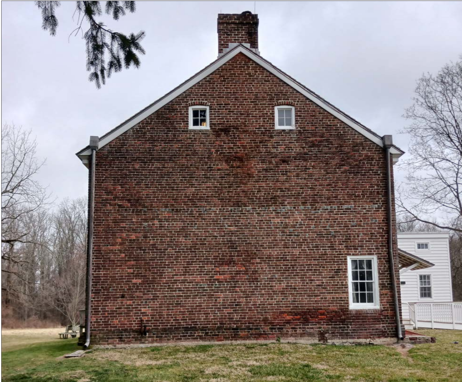
55-1: West elevation of the house.
