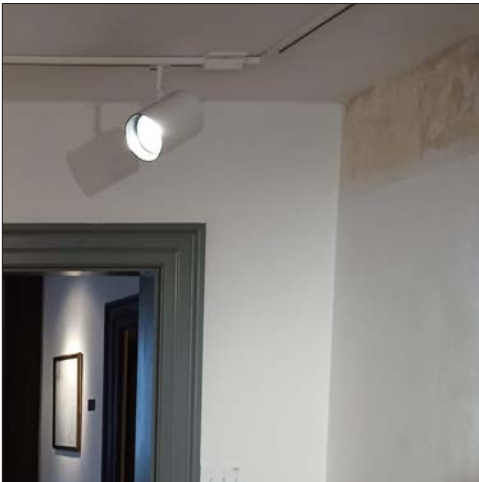
82-2: Previous investigations of the interior finishes revealed stencil work.
