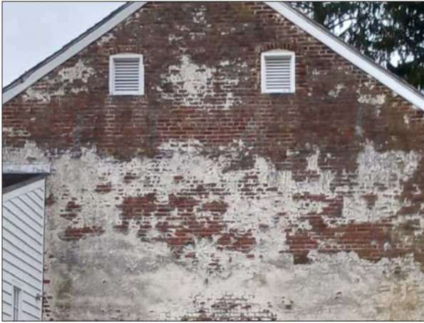
136-1: Upper East gable end featuring '1761' in vitrified brick.
