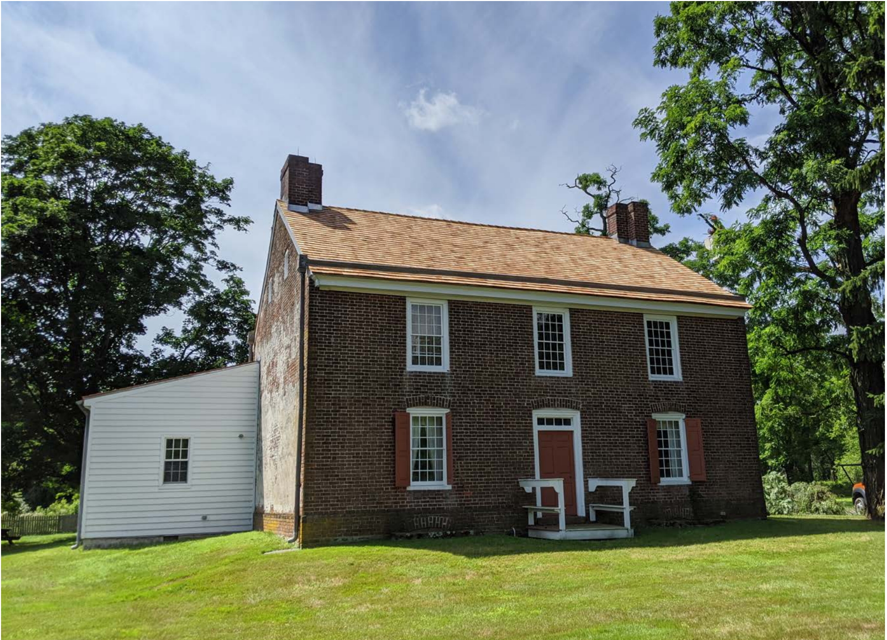
9-1: Northern facade of the house.
