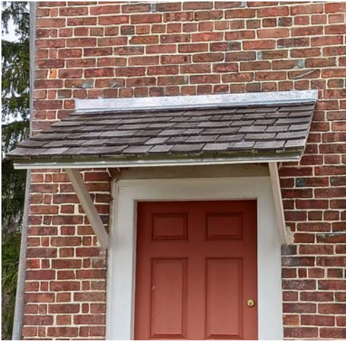
46-1: Shed roofs over doors at South elevation.
