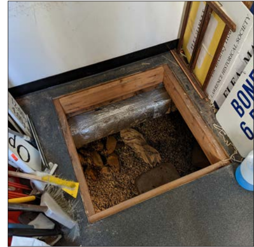
85-3: Crawl space access from inside of closet.
