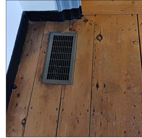
73-5: Floor-mounted mechanical register cut into original flooring.
