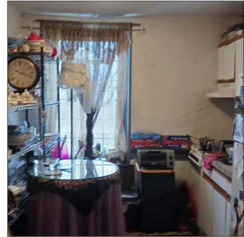
91-3: Existing conditions of the window and plaster at the tenant kitchen.
