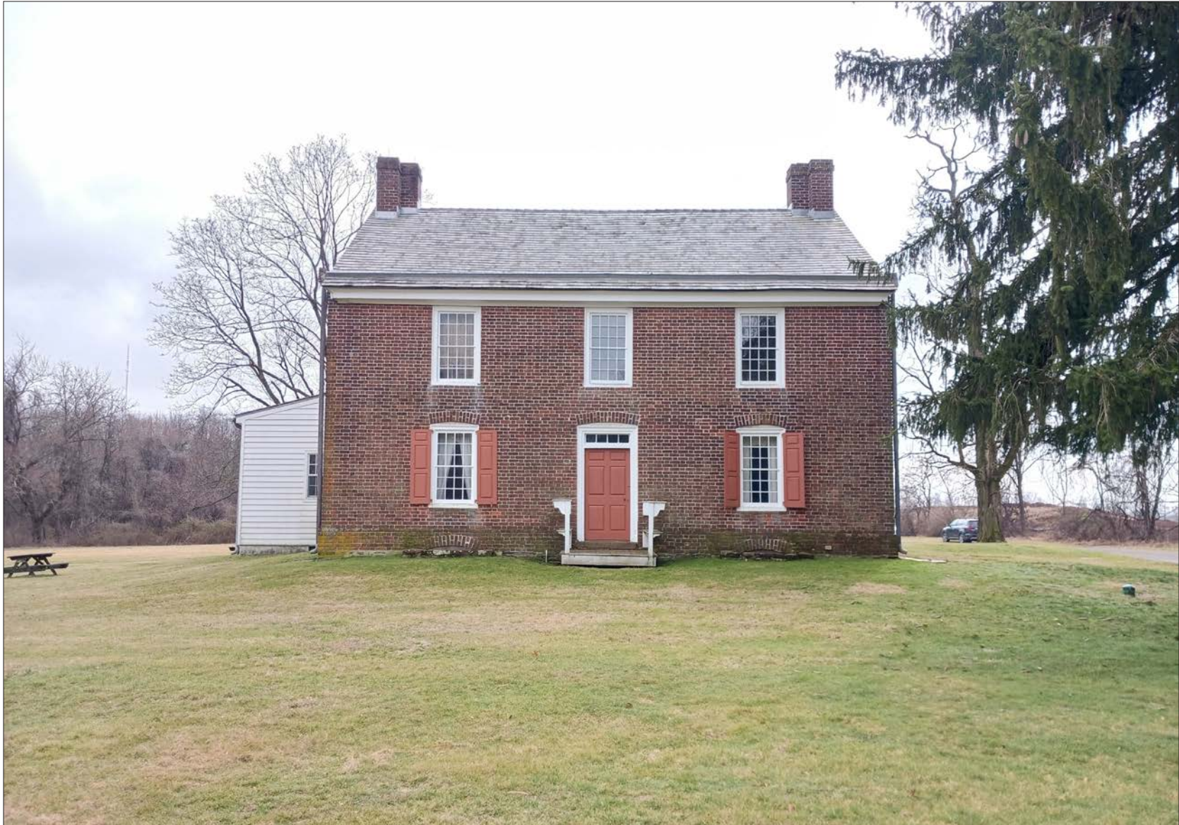
105-1: The building is a multi-wythe brick masonry wall bearing structure,
