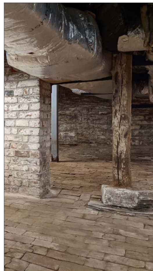
103-1: View of basement showing wood, brick, and steel structural columns.
