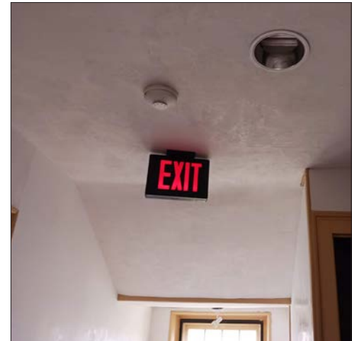
87-3: Second floor corridor ceiling has contemporary lighting and safety equipment.
