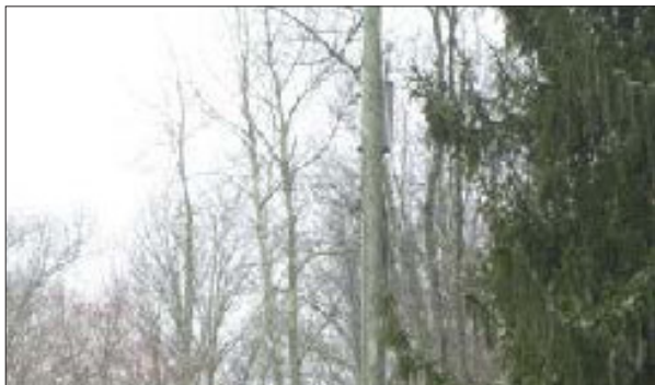
110-2: Fig. E-1 25 kVA transformer
