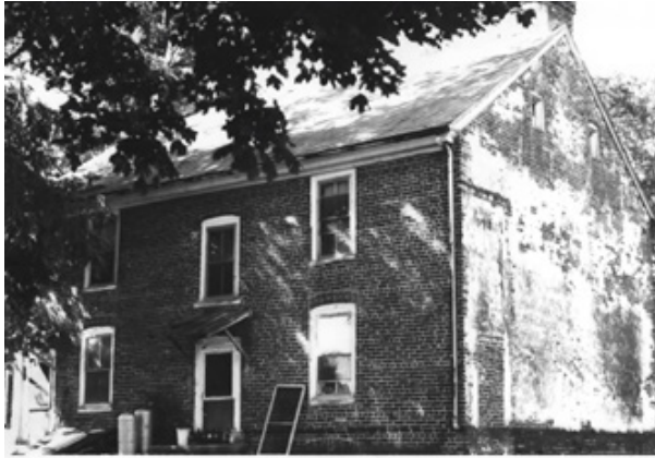
Figure 2: The asymmetrical rear elevation in 1979. Gottuso, Baker-Brearley House Nomination.
