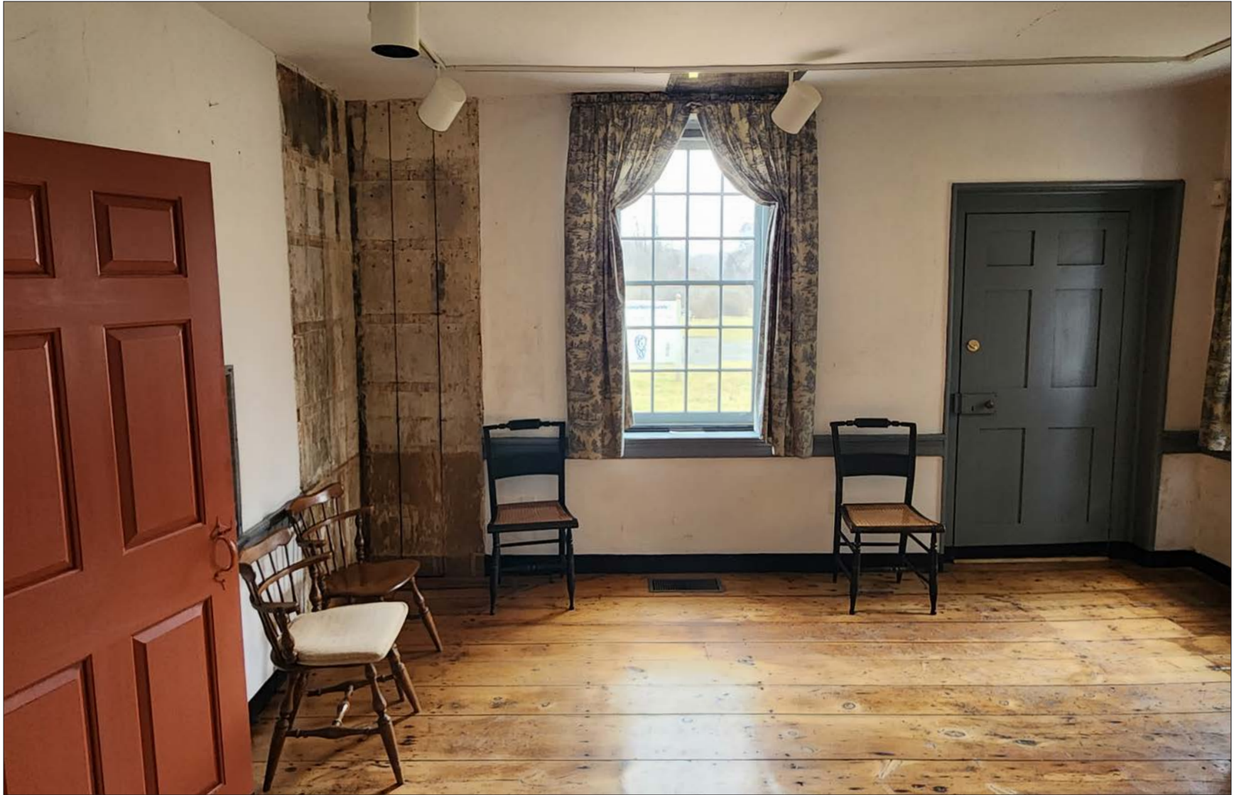
75-1: This room uses the investigation into historical finishes and construction as an interpretive tool.
