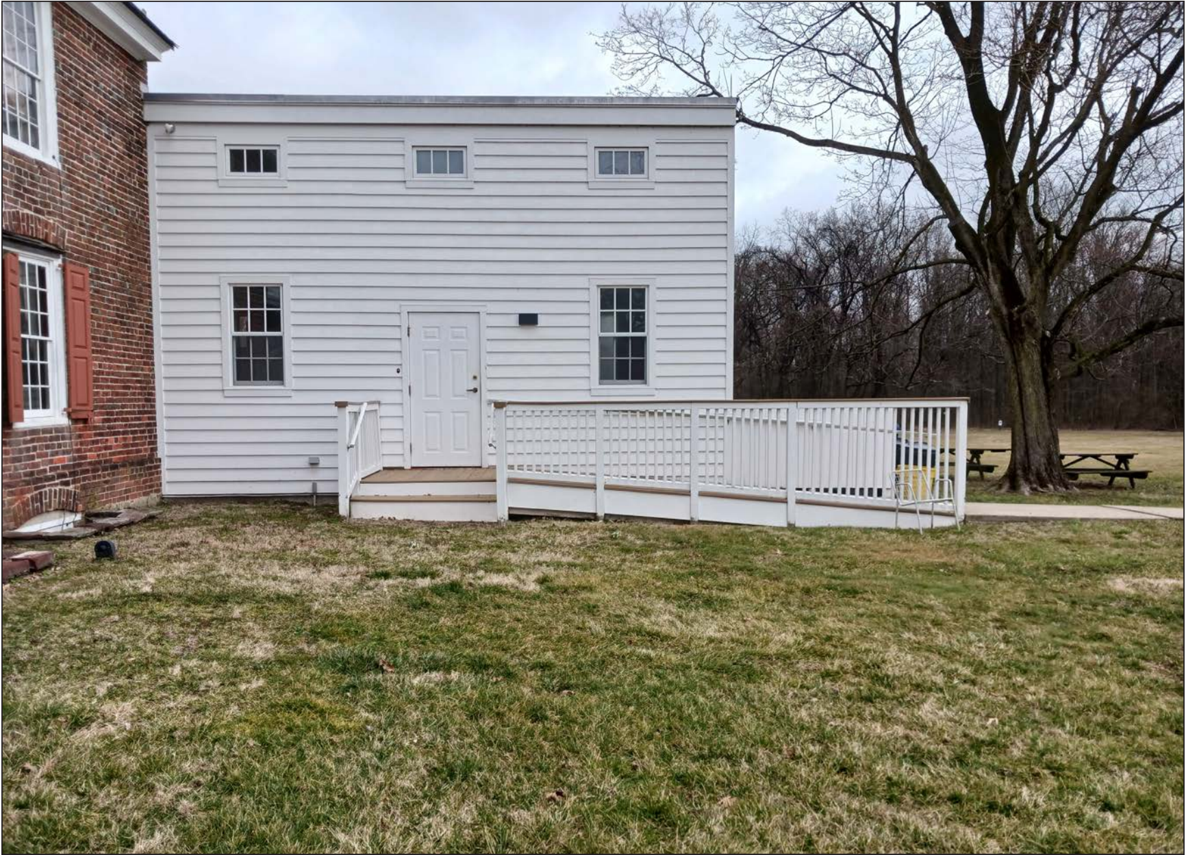
57-1: West elevation of addition showing accessible ramp and steps.
