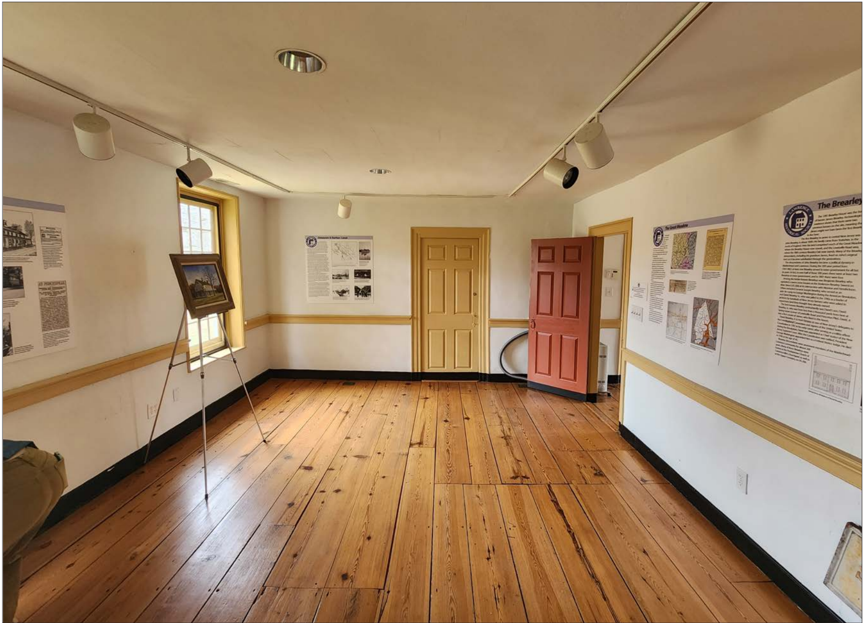
99-1: Original floorboards, closets, and frame are original and should be maintained.
