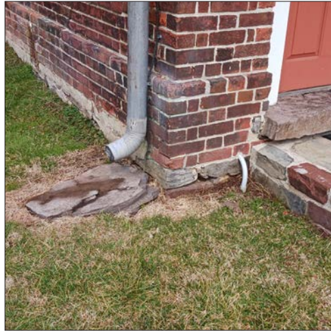
46-2: Existing downspout and foundation
