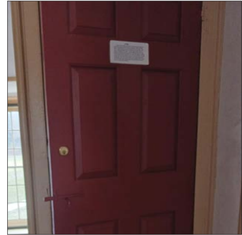
87-2: Door to attic
