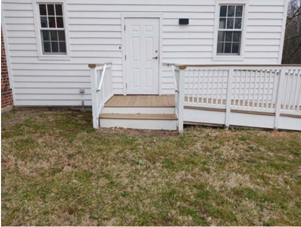
142-1: The addition provides an accessible entrance and necessary public restrooms.
