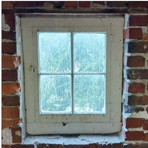
101-3: Typical attic casement window.
