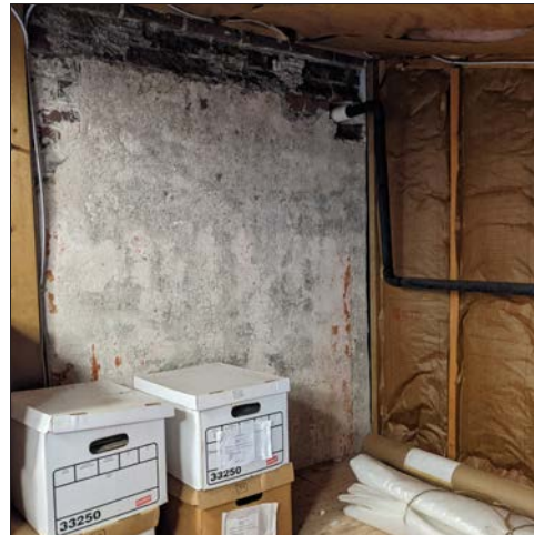
85-5: Storage space above Kitchen wing showing connection to brick wall.
