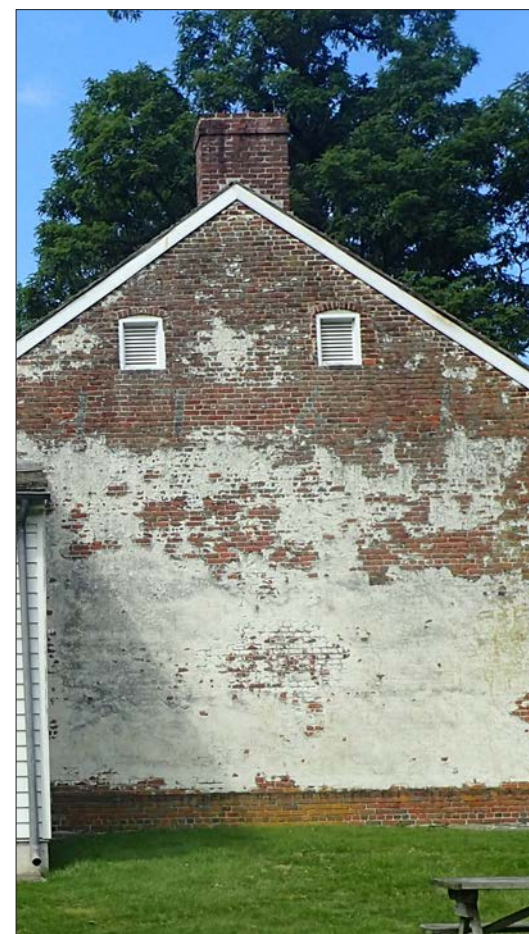
15-1: East gable elevation, showing ‘1761’ in vitrified brick.
